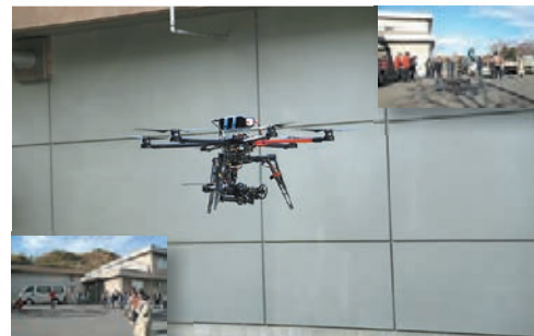
Bridge inspection using a multicopter
