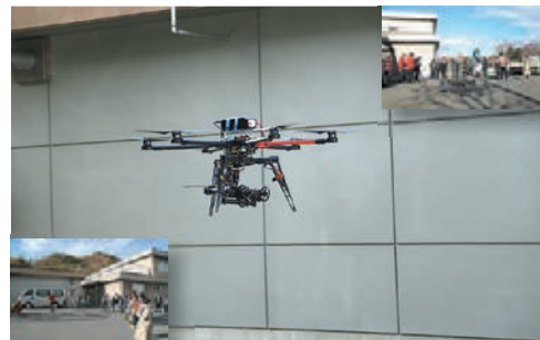
Bridge inspection using a multicopter
