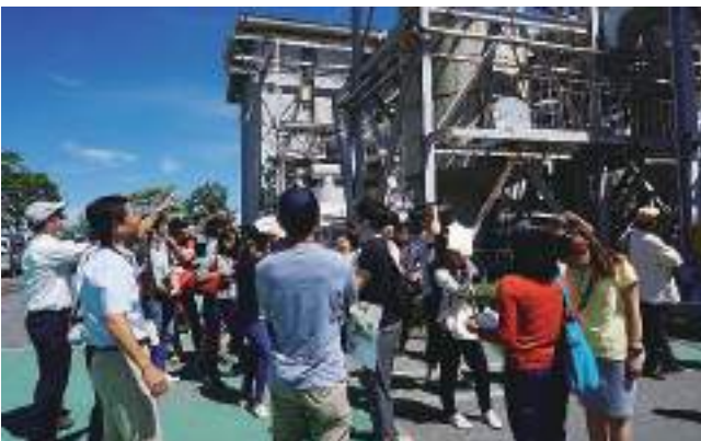
Geothermal Electric Power Plant, Beppu City, Oita
